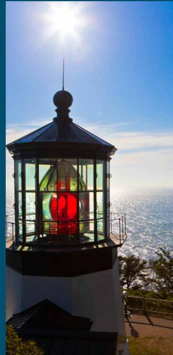
Oregon's shortest lighthouse stands 38 feet atop Cape Meares and 217 feet above the ocean. In January 1886, the U.S. Congress approved \$60,000 for construction of the lighthouse, which later took one year to build. Craftsmen built the tower using bricks made on site and then covered the exterior with iron plates.
